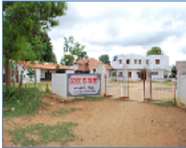
View of VGHS School Classroom
